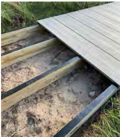
Add joist tape for protection
