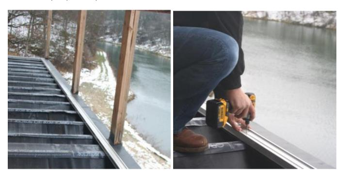
**Step 6:** Using a single tile as a spacer, place the tile groove over the male spline on your starting track. Place several tiles along the length of your track piece, these will serve as a guide for your next 2-sided track.
