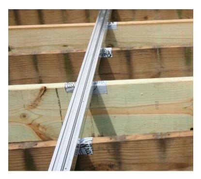
**Step 5:** Place a single sided rail per your layout at your designated starting edge. Once you have positioned the track piece, pre-drill a hole using a 3/16" drill bit at all points where the rail will intersect the deck joists. Secure track to joist using stainless screws provided. Snug securely, do not over tighten causing track to warp. Make sure the track stays square to your deck.
