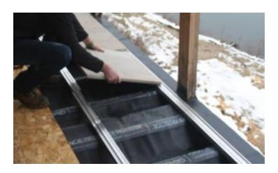
**Step 8:** Move any of your spacer tiles as necessary to place screws. Install all tiles in that row before starting on next. A rubber mallet may be used for sliding the track into the machined groove in the tile. Always check for square and parallel to structure and finish row.
