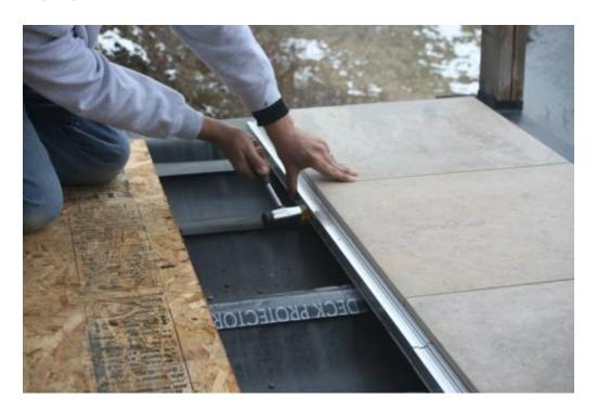
**Step 9:** Repeat steps 1-8 until last row then using a single sided track at edge slide final row of tiles in from end.
