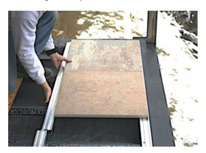
**Step 7:** Lift the tile sliding the next track into place sideways. Align your pre-drilled holes to your deck joist. Install 1 screw at each joist securely but not over tightened.
