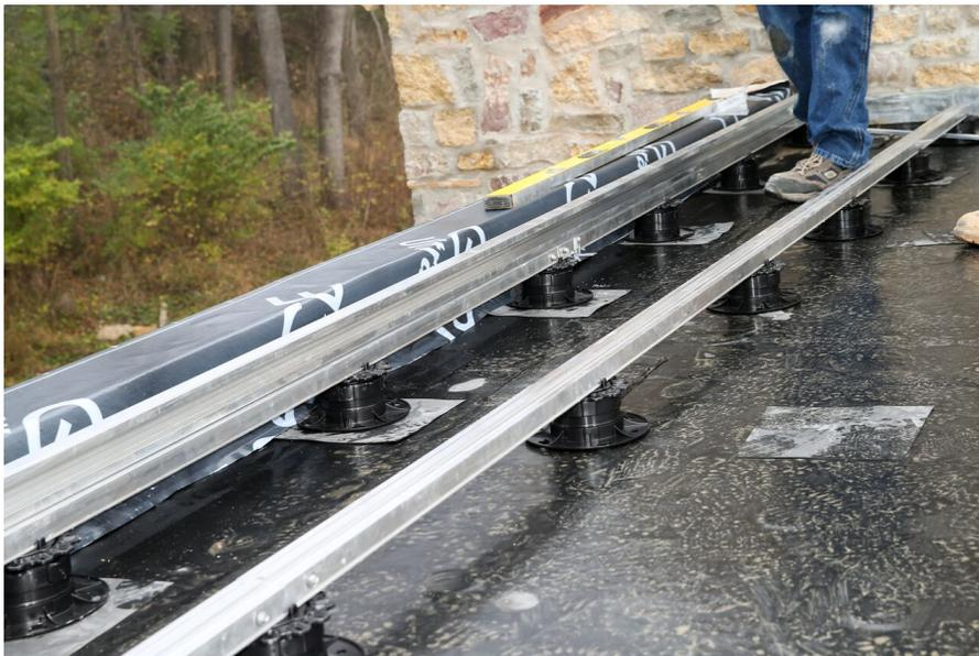
**Step 7:** Once tile layout is figured, use supplied epoxy adhesive to fasten tiles. Apply half-dollar-size amounts every 6 inches to top of perimeter track. DO NOT APPLY ADHESIVE DIRECTLY TO WATERPROOF MEMBRANE.
