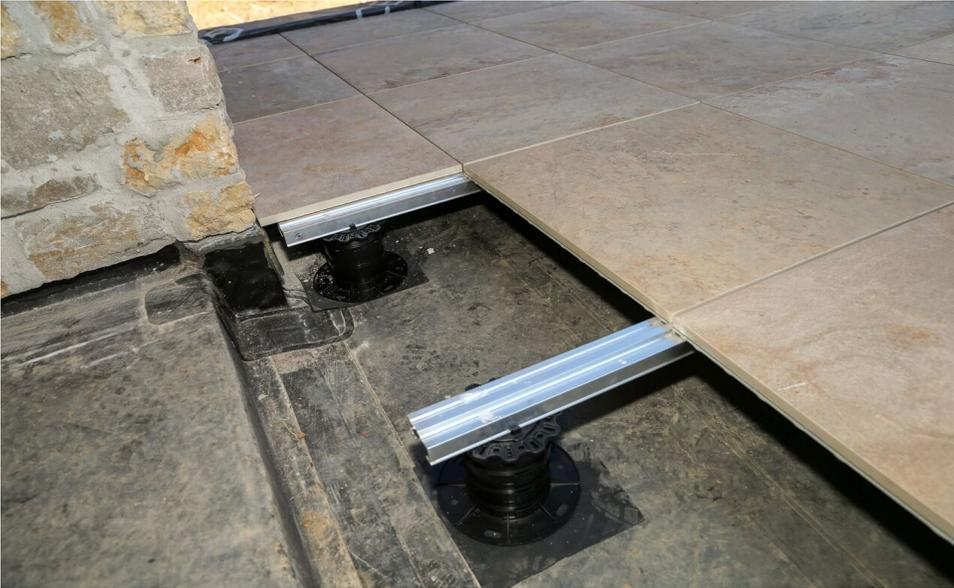
**Step 18:** Use Mbrico perimeter flat track to finish final row against structure. A 1/8" gap should be left between Mbrico surface edge and any structure or wall to allow for proper drainage. See step 7.
