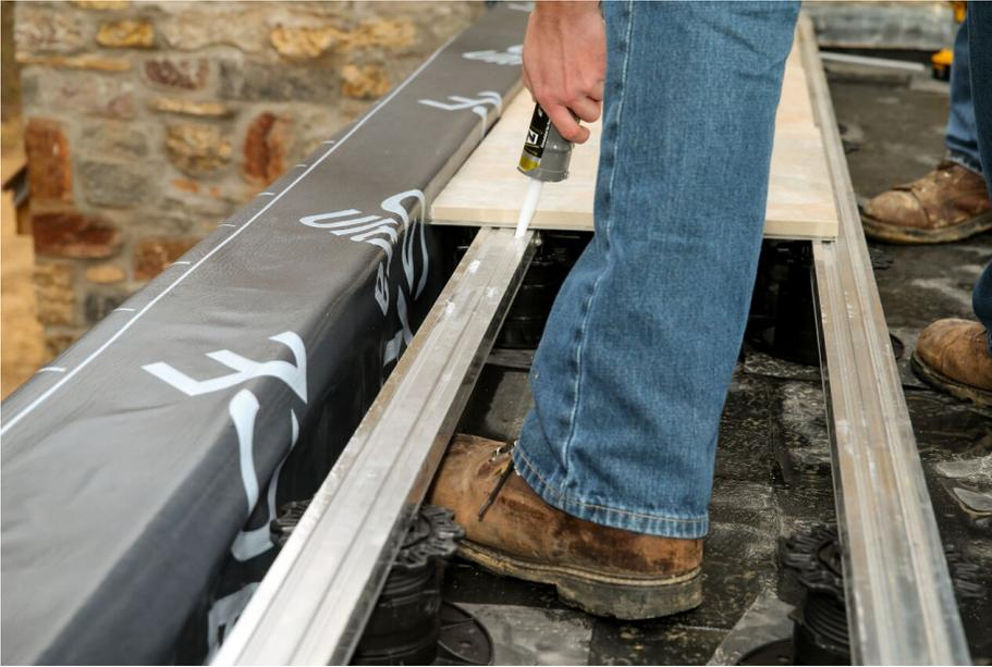
**Step 8:** Tiles are to be adhered to perimeter track and overlap to compensate for distance between wall and pedestal. Leave at least 1/8" gap between tile and structure.
