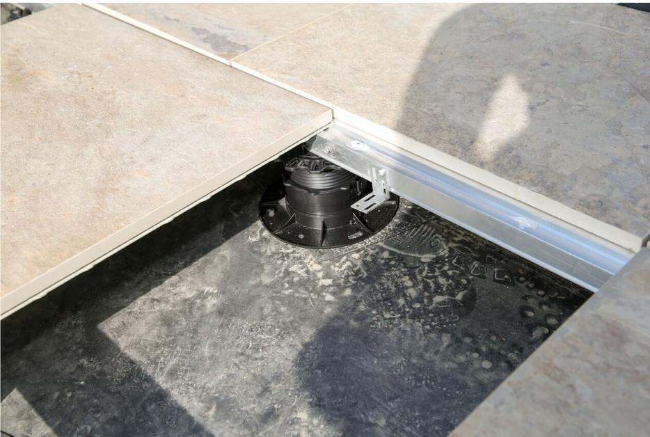
**Step 11:** For non-perimeter rows, use and Mbrico T-Track so tiles can be received on both sides of the track. This provides automatic spacing and captures the tiles.
