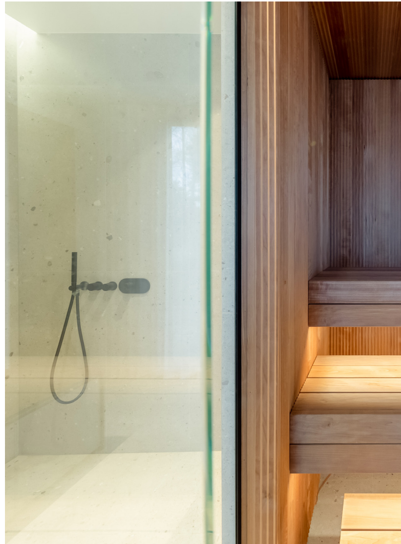
Walls & Ceiling: Medium Modified Aspen Vire, Bench: Medium Modified Aspen SHP. Private Home, Estonia. Photo by Elvo Jakobson
